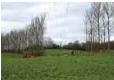
Clearing an 11kV Line through a line of Poplars ( Populus spp )
