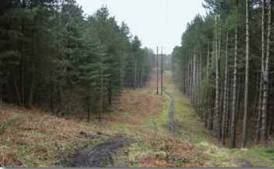
A 33kV overhead line through a commercial forestry plantation
